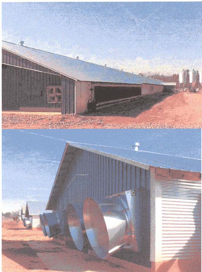
Figure 1. Broiler production house: Top is evaporative cooler end, bottom is tunnel fan end.
